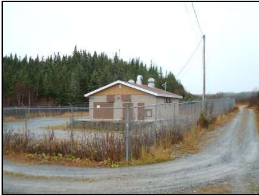
Figure 8. Water treatment facility at Trout Pond (photo by Adam Anderson).
