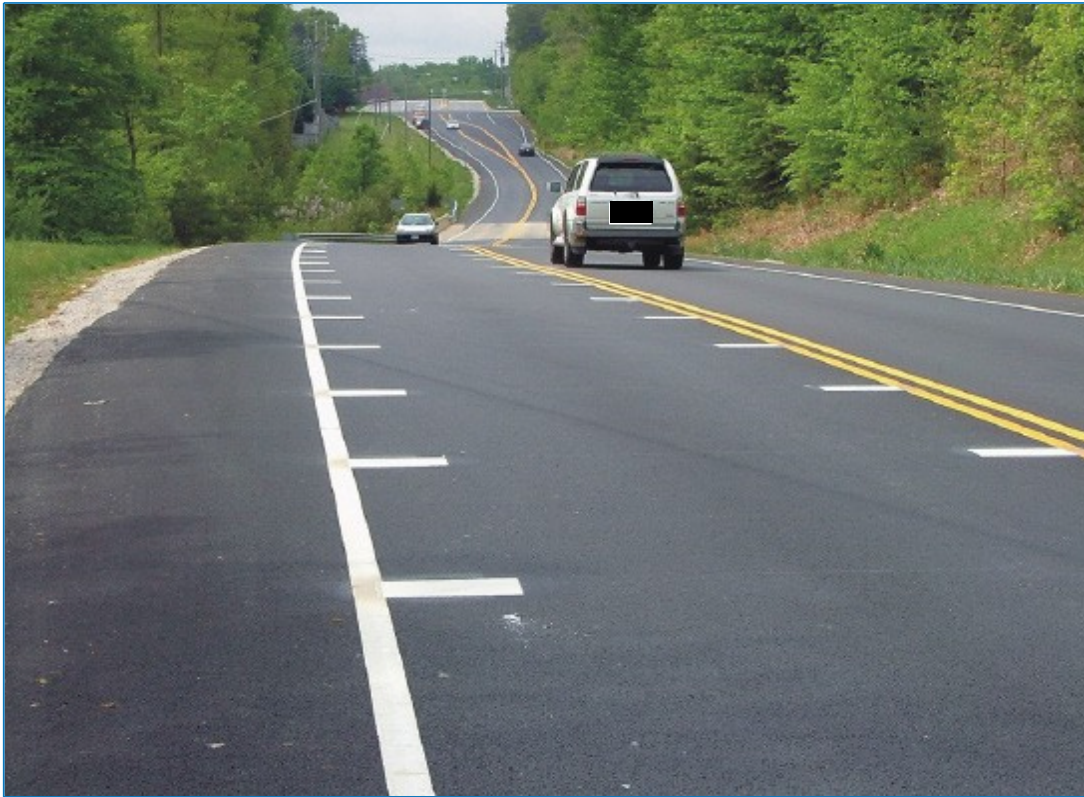
Figure 25: Peripheral Transverse Bars - Image Source: FHWA
