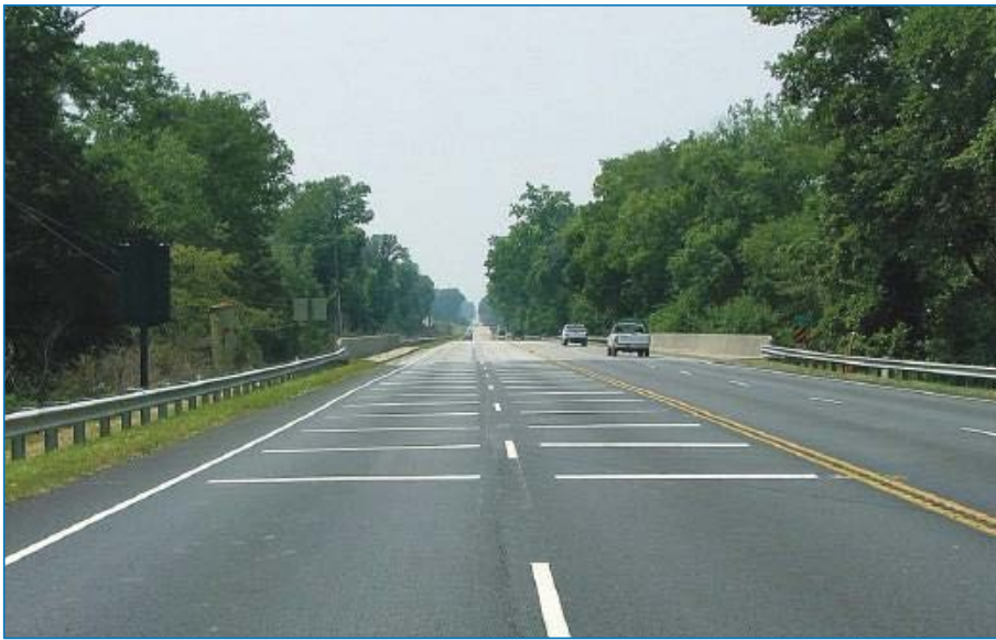
Figure 24: Full-Lane Transverse Bars - Image Source: FHWA
