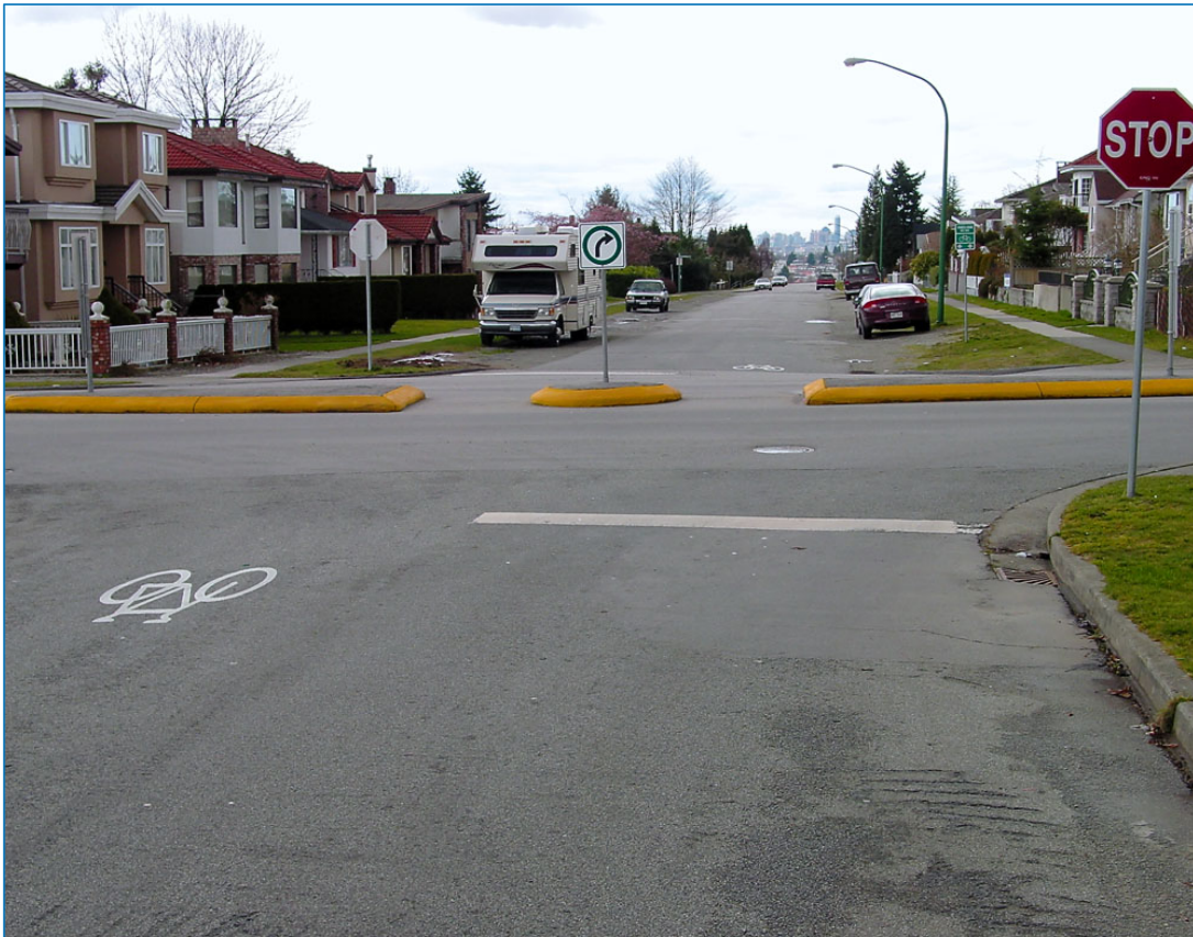
Figure 31: Raised Median Through Intersection - Image Source: Richard Drdul
