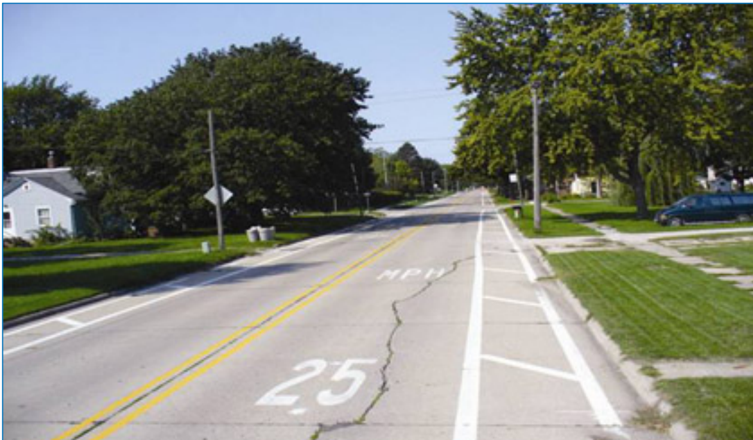
Figure 13: Lane Narrowing - Image Source: FHWA
