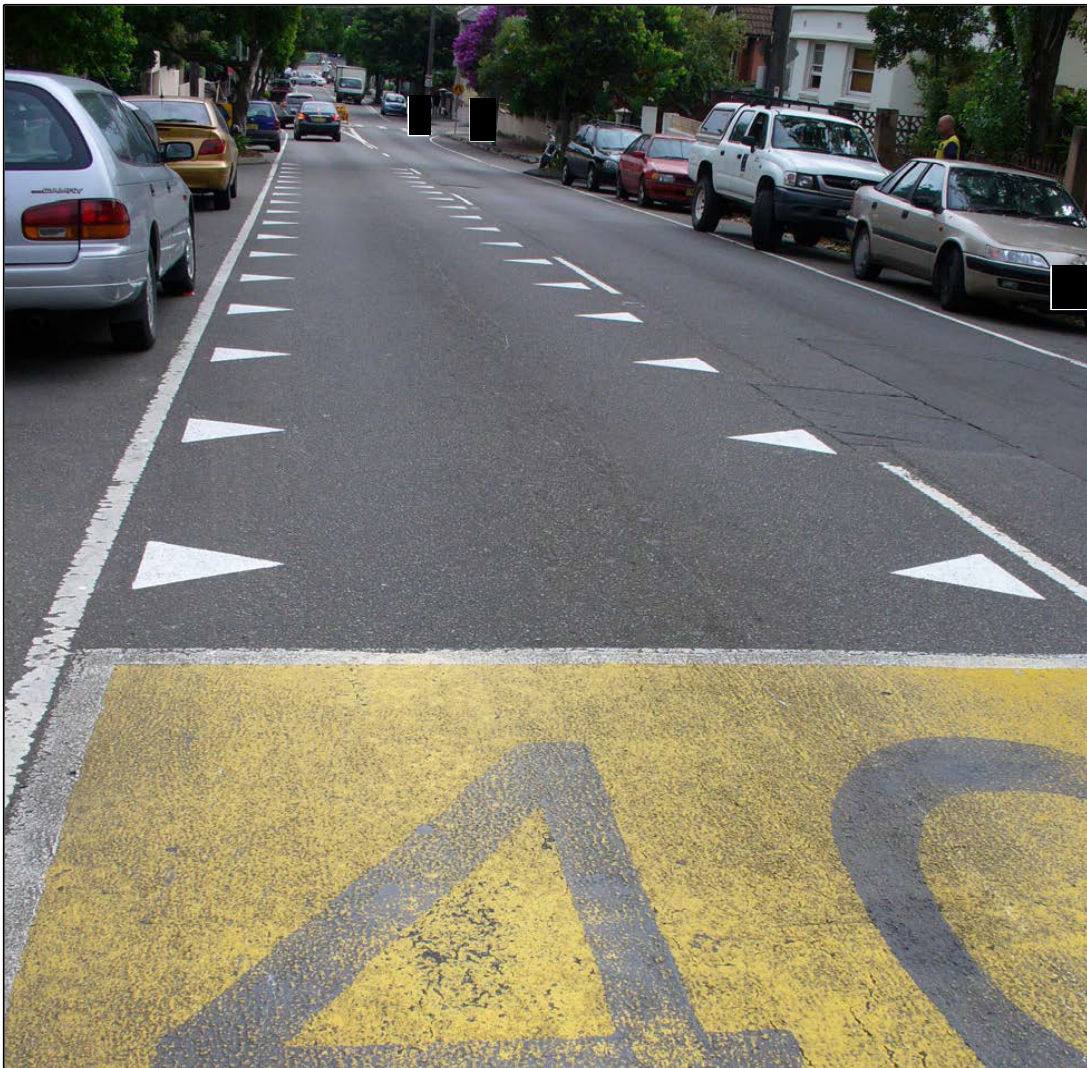
Figure 23: Dragon's Teeth - Image Source: meganix.net/pavement
