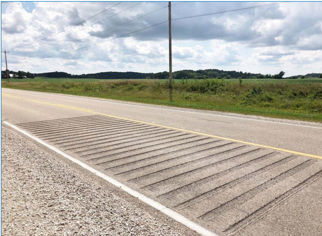
Figure 21: Transverse Rumble Strips - Image Source: Journal Times
