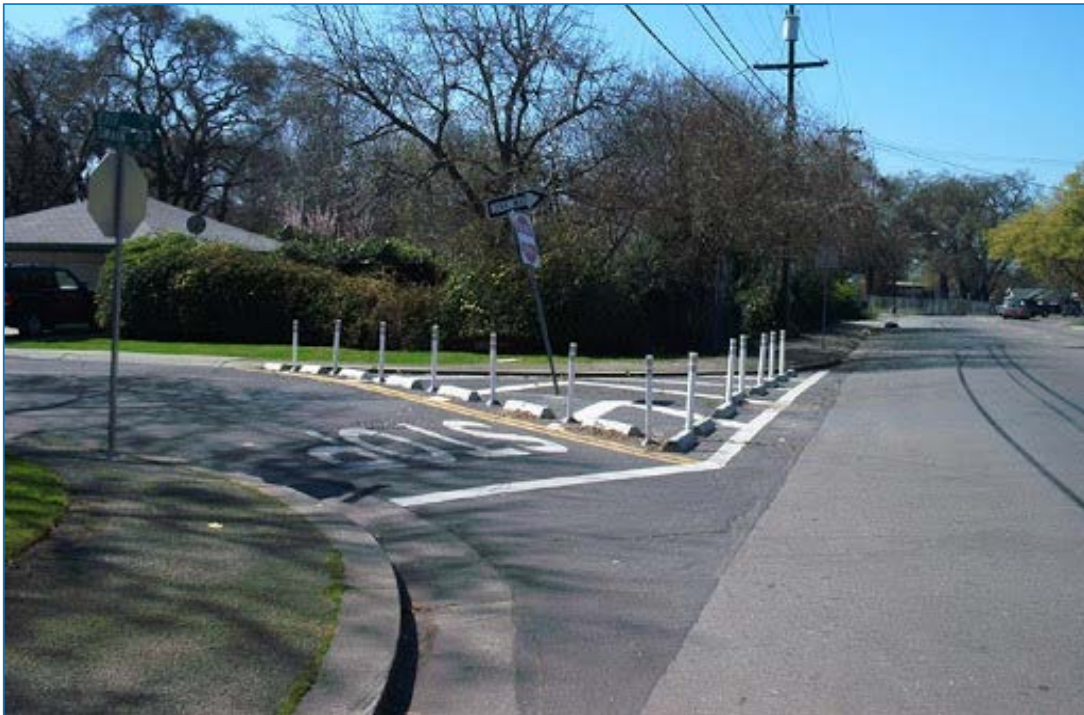
Figure 30: Intersection Channelization - Image Source: City of Stockton
