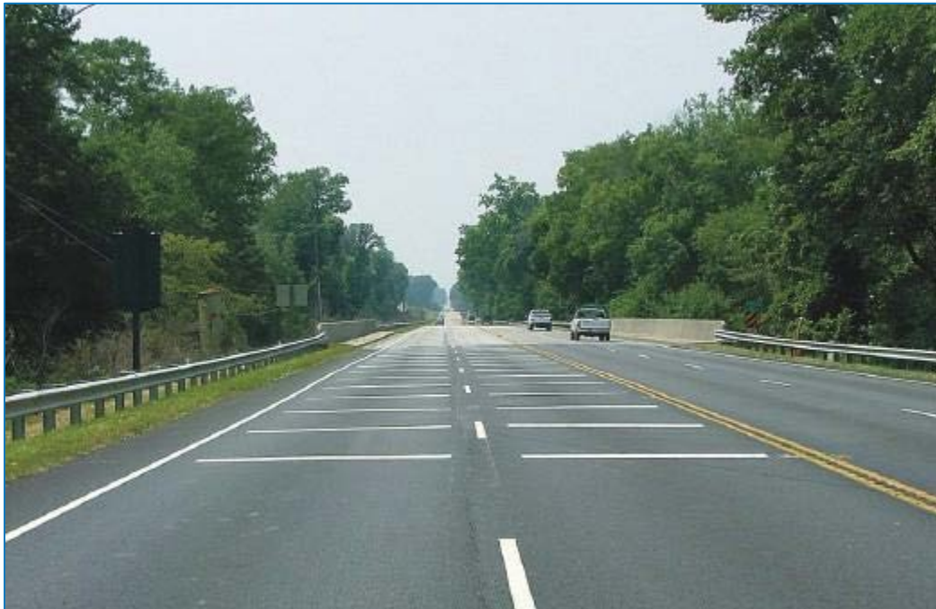
Figure 24: Full-Lane Transverse Bars - Image Source: FHWA
