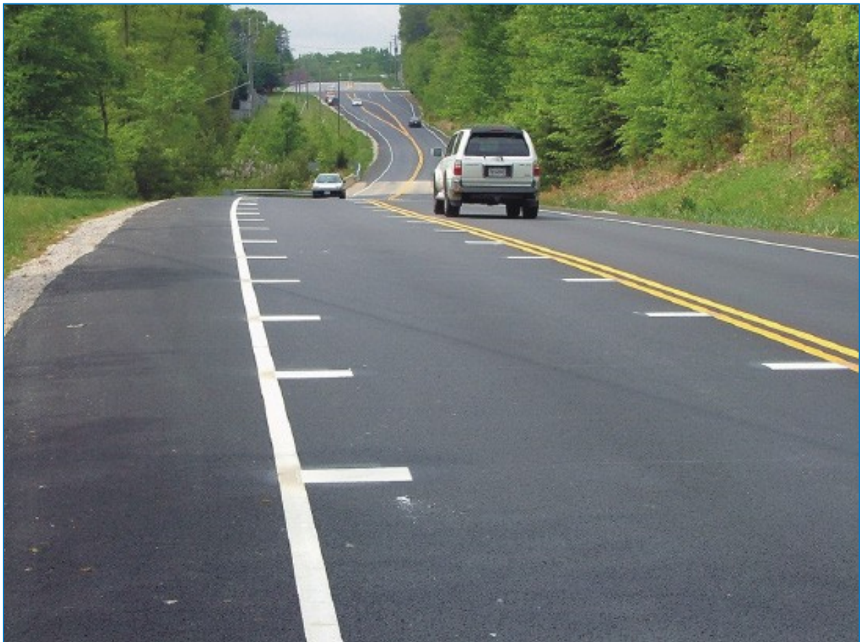
Figure 25: Peripheral Transverse Bars - Image Source: FHWA
