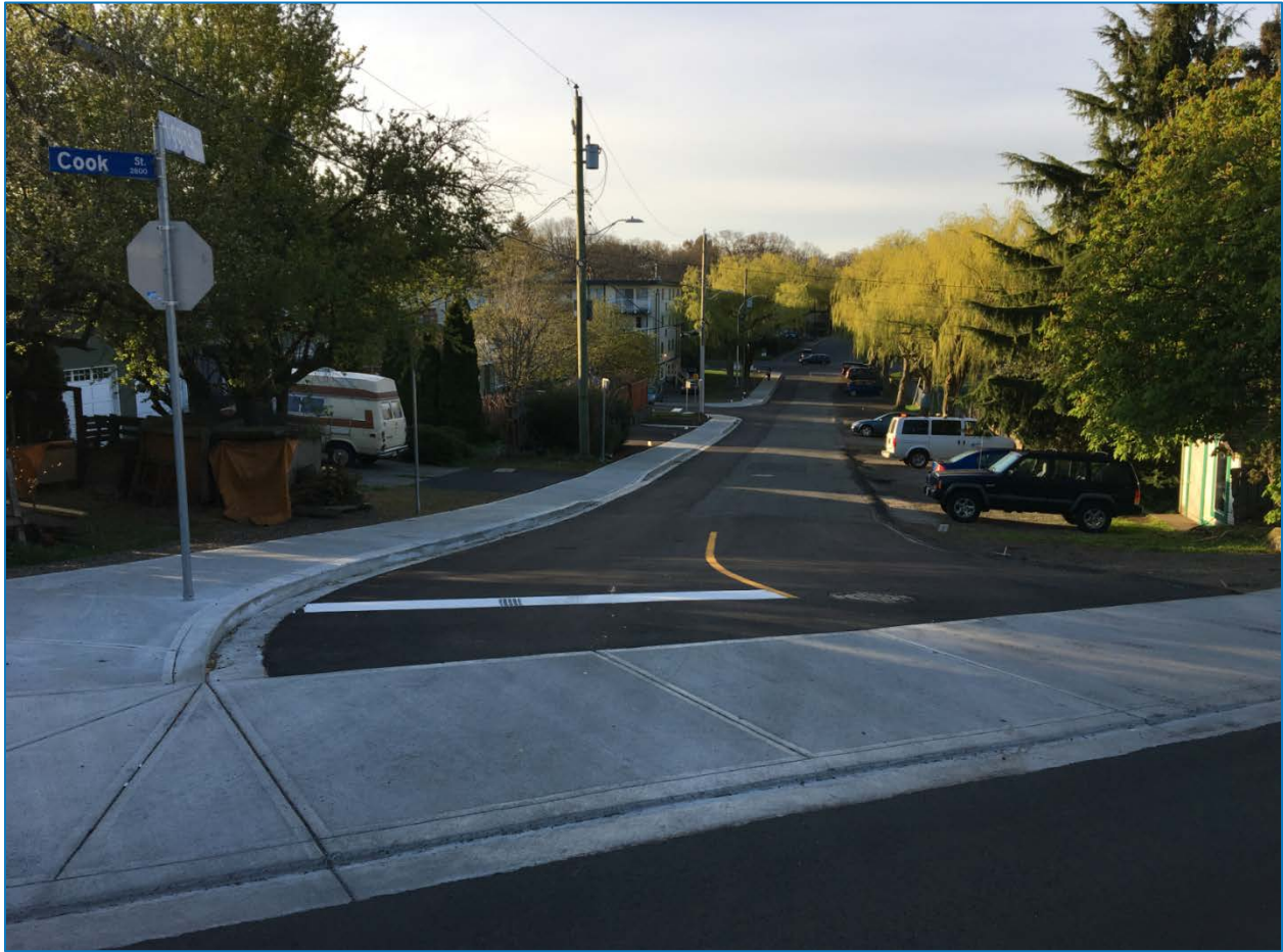
Figure 19: Sidewalk Extension - Image Source: City of Victoria
