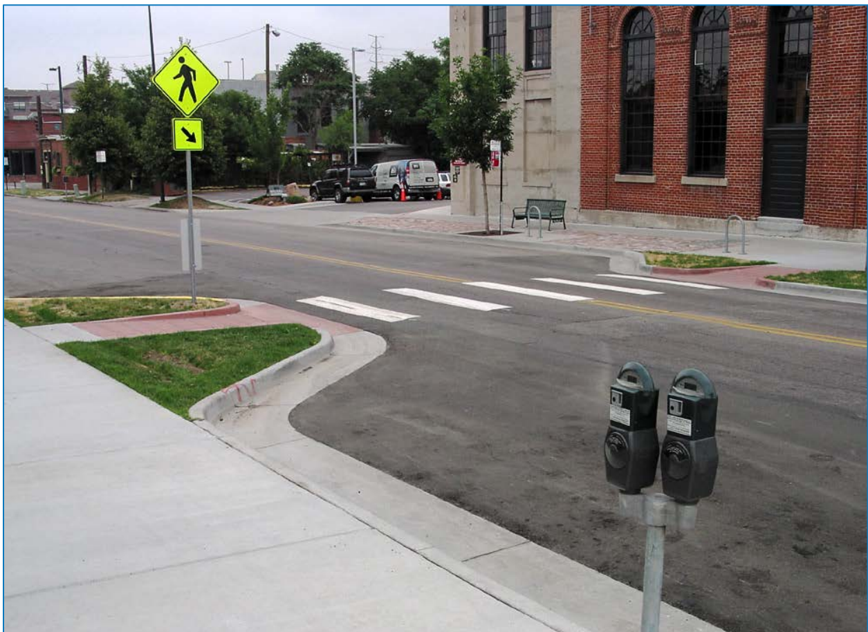
Figure 12: Curb Extension - Image Source: Richard Drdul
