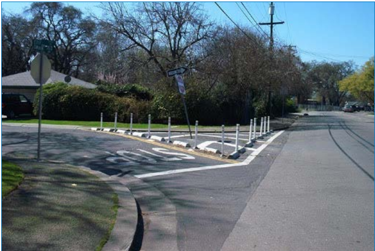
Figure 30: Intersection Channelization - Image Source: City of Stockton
